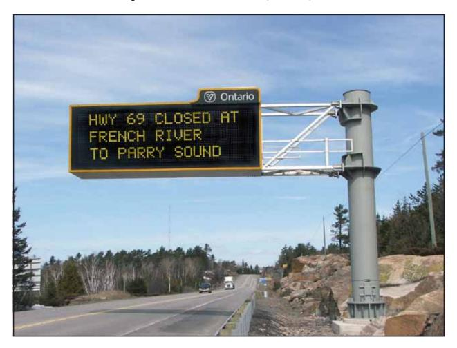
Figure 8 – MTO Roadside-mounted (Cantilever) VMS
